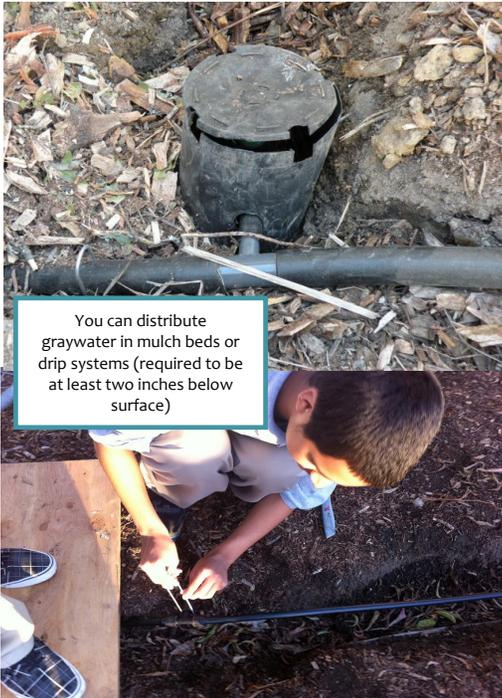
Example of valve that allows user to switch between irrigation zones
